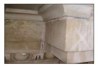
In almost all circumstances, only Impressed Current systems can be shown to provide the level of protection required. Masonry is generally drier than soil or concrete requiring high drive-voltages to deliver and distribute the protection-current. Galvanic systems [including the galvanic stage of hybrid systems] are usually unable to generate the voltages needed to pass current through the masonry to areas remote from the anode.
